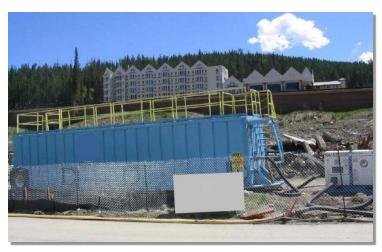
**Photograph CT-1.** Proprietary chemical treatment system being used on a construction site with sensitive receiving waters. Photo courtesy of WWE.
